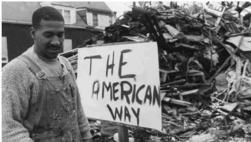
Tyree Guyton looks at the demolition of his work on Oct. 24, 1991. Detroit Mayor Coleman Young, responding to neighborhood complaints, ordered three of his houses bulldozed.
