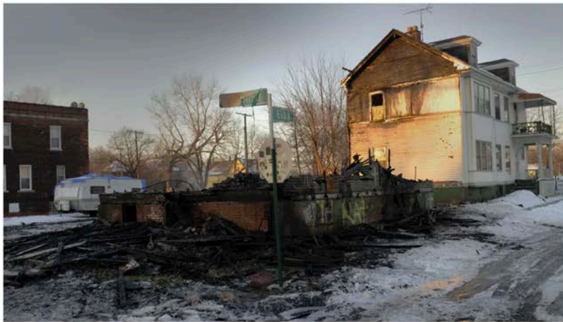
The Party Animal House, also known as the Doll House, burned to the ground on March 7, 2014.
